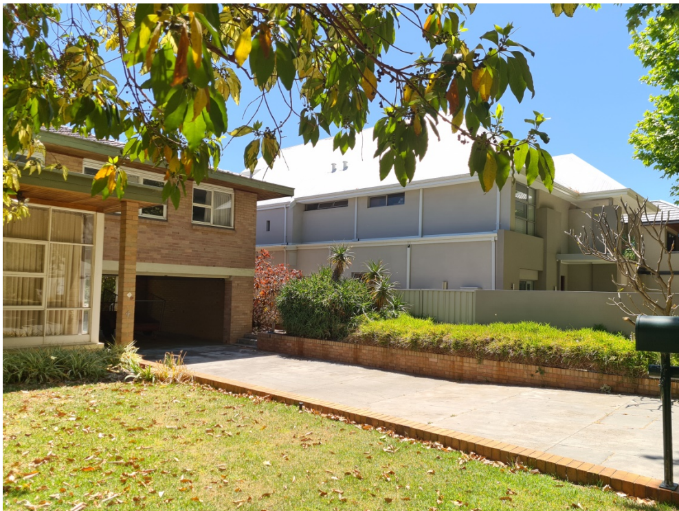
Figure 14: View east to the existing home at 2B Tweeddale Rd, noting absence of major openings.
