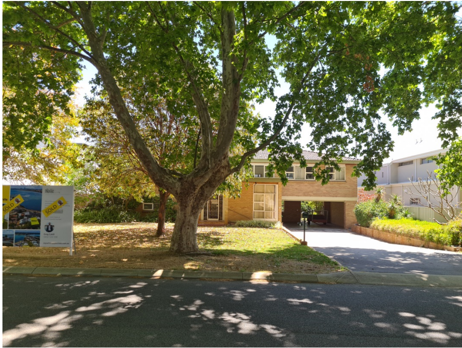
Figure 13: View north of the existing dwelling from Tweeddale Road. The tree seen in the foreground is to be retained
