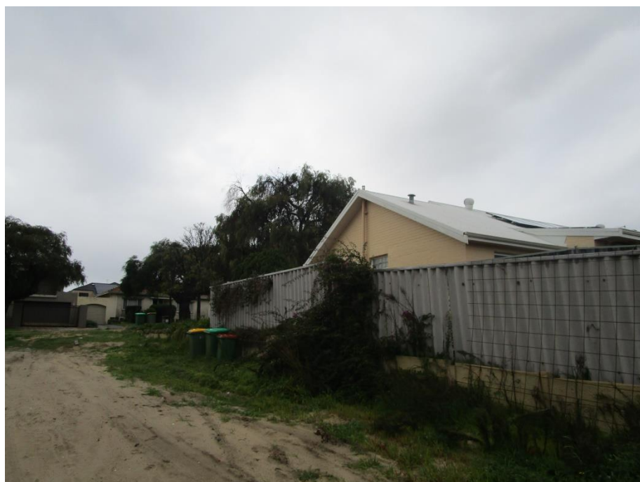
Figure 9: View south east to the dwelling at 38 Raymond Street. The access leg servicing 38A Raymond Street is behind the super six fence.
