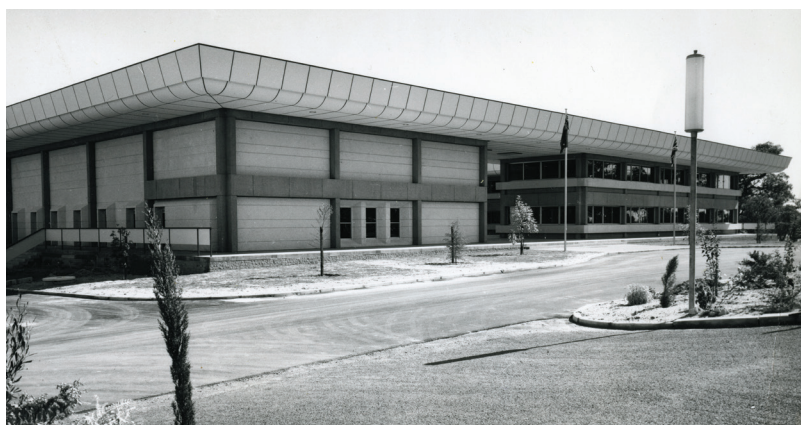
The Melville Civic Centre was opened on Wednesday, 1 May 1968
