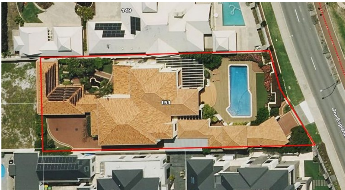
Figure 1: Aerial photography of subject site.
