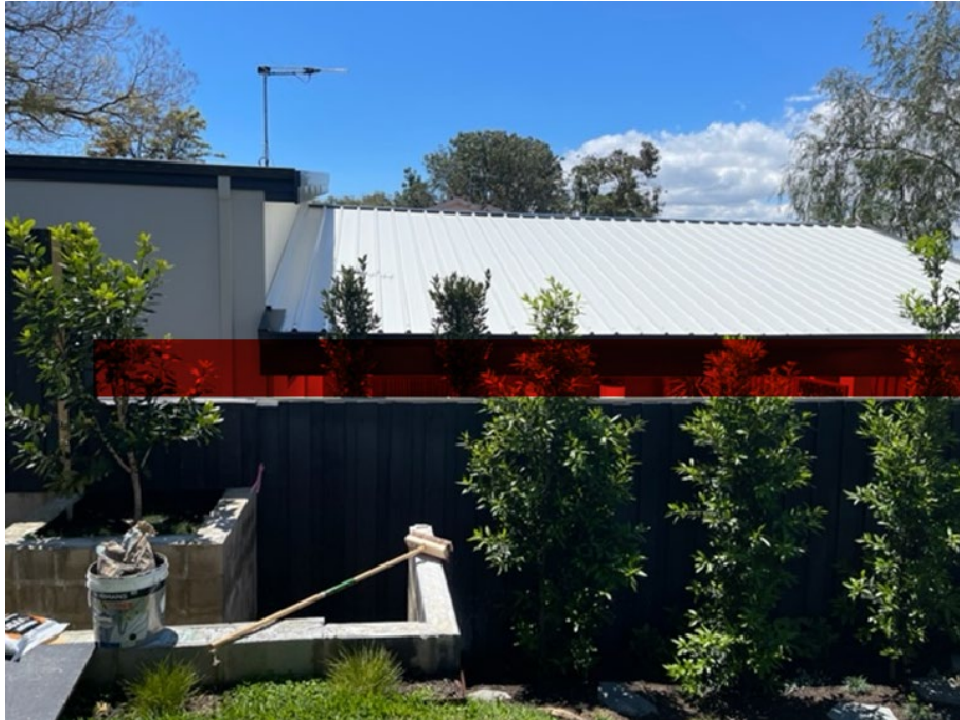
Figure 3 – Proposed location of screen wall from viewed from the subject site. The red block indicates the location of the proposed screen structure.
