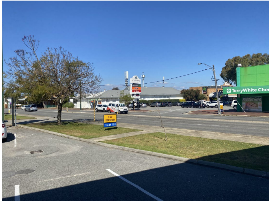
Figure 2 – View of the existing monopoles on the Telstra exchange building
