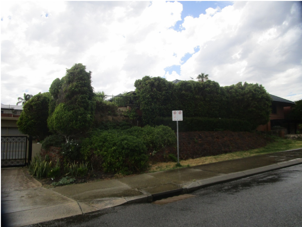
Figure 9: Area of retaining and fill which is to be removed within the verge and front setback on the western boundary
