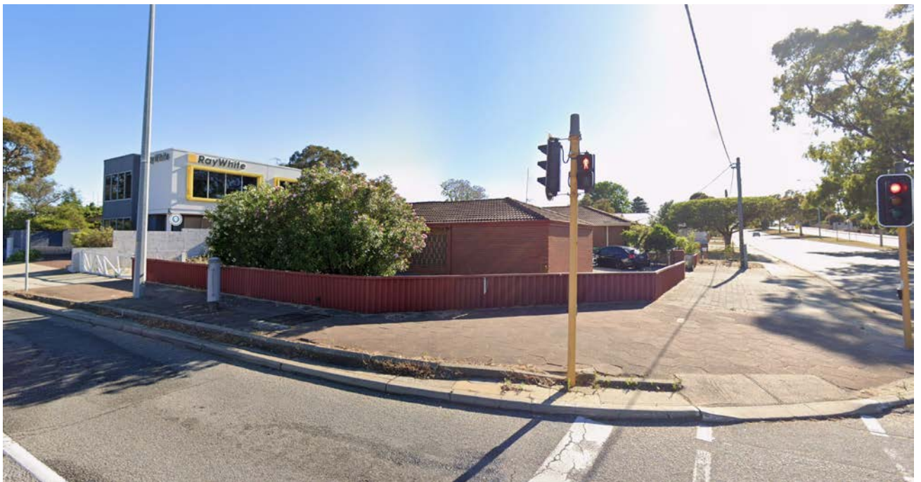
Figure 4 East Facing of Subject Site
