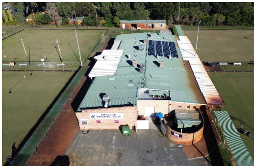
Aerial view –Main building
