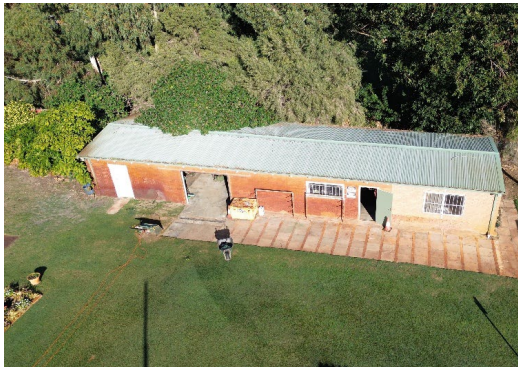
Aerial view –Groundsman's shed
