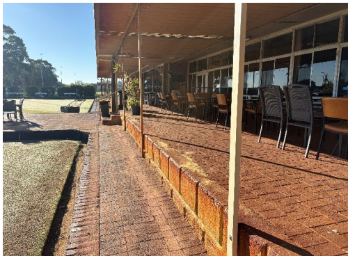
General view verandah
