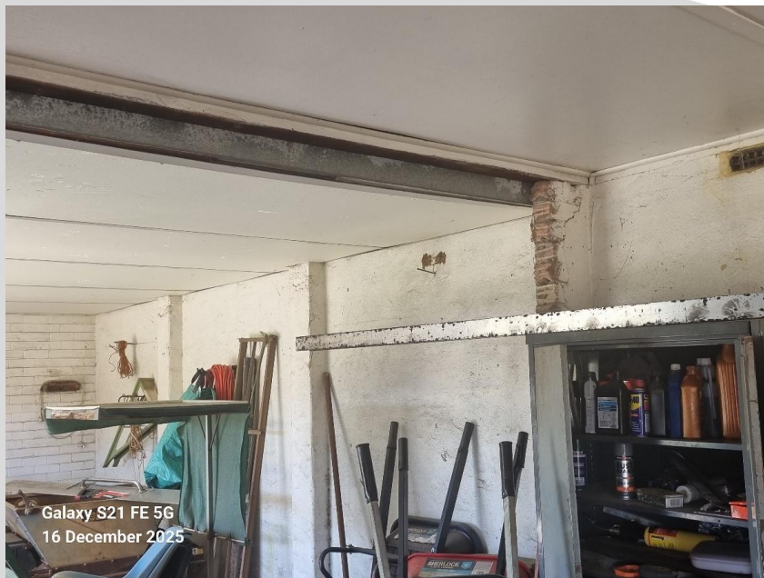
25. INTERNAL PARTISION WALL – Wall has been removed
