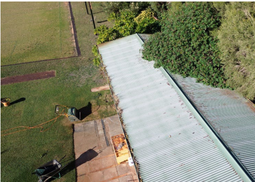
Aerial view –Overgrown vegetation
