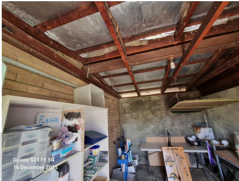
24. TYPICAL ROOF STRUCTURE – Good condition
