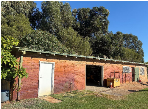
Groundsman's shed – General view
