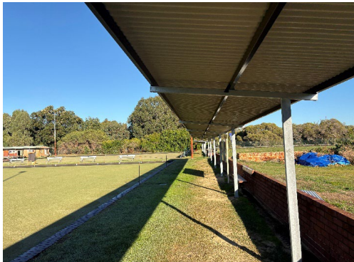
General view new shade structure
