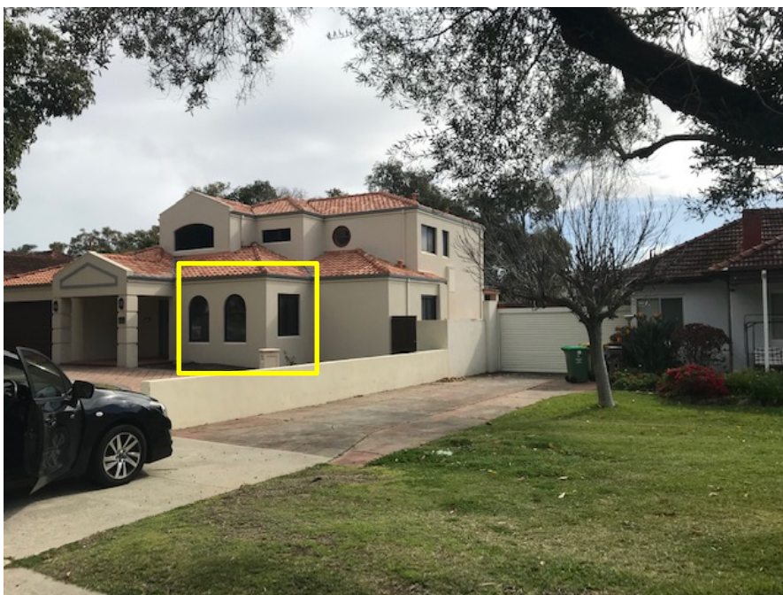
Figure 3: Close up view of the neighbouring property. The windows highlighted in yellow will have an oblique view of the non-conforming section of wall.
