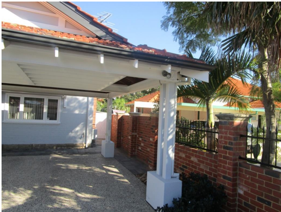
Figure 3: View of the neighbouring property's carport and driveway area. The proposed garage parapet wall will be located abutting this area.
