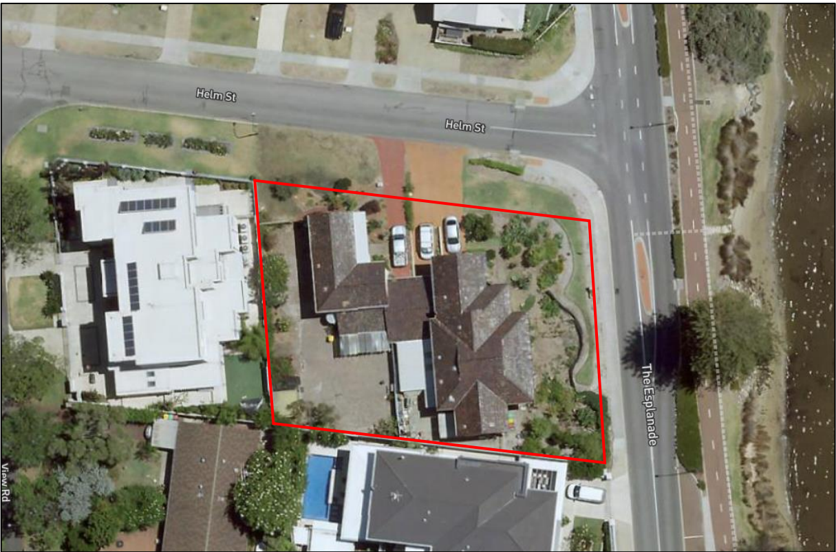
Figure 2: Aerial View (December 2020)
