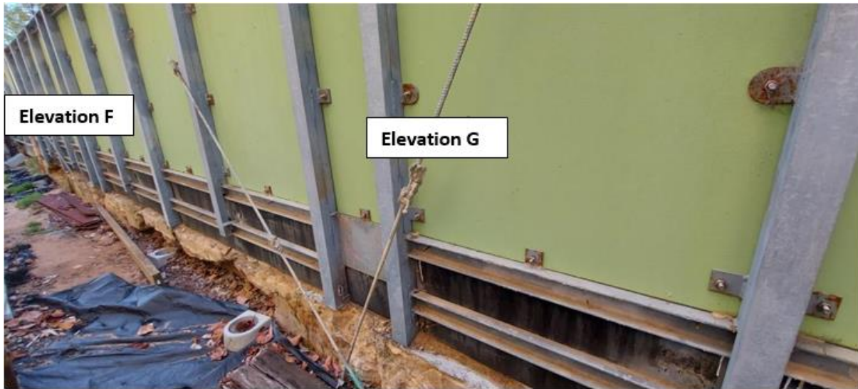
Photo 6 shows Elevation F & G
