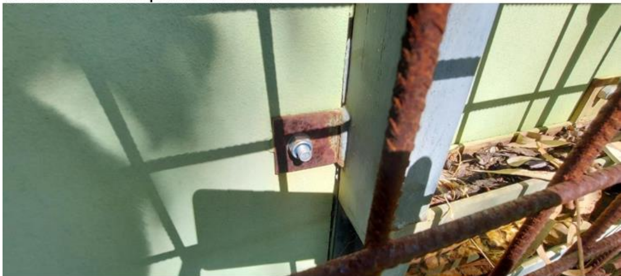
Photo 4 shows sheet connection
