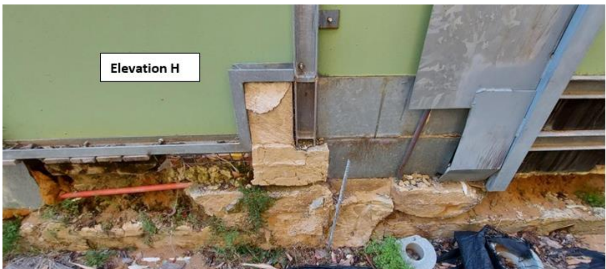
Photo 5 shows Elevation H
