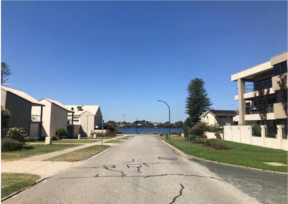
Photograph 4: View of Helm Street facing east with the subject site on the right hand side.
