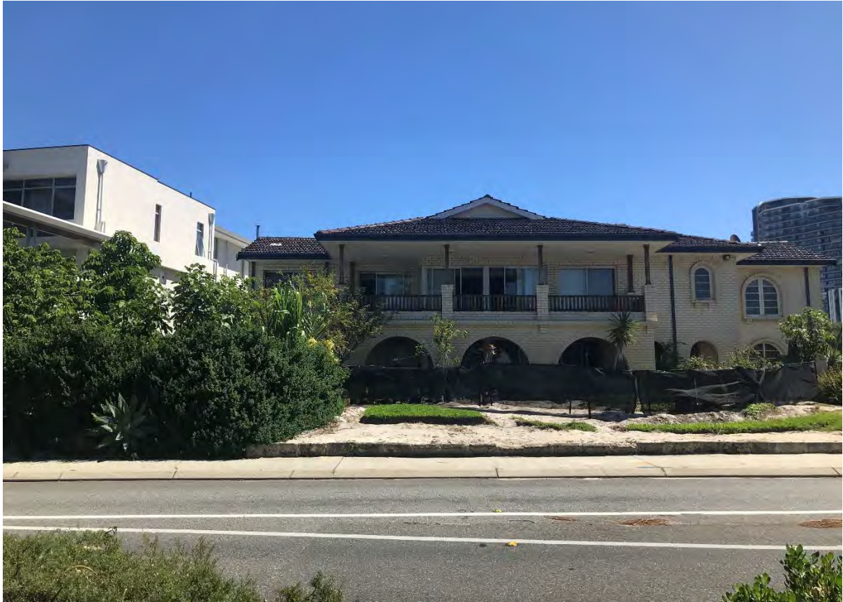
Photograph 8: Subject site as viewed from the opposite side of The Esplanade
