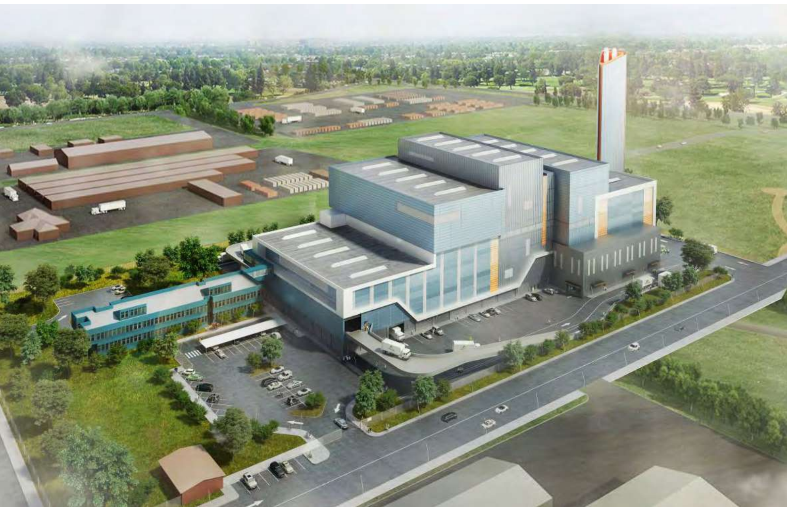
Avertas Energy's 'Waste-to-Energy' project currently under construction in Kwinana
