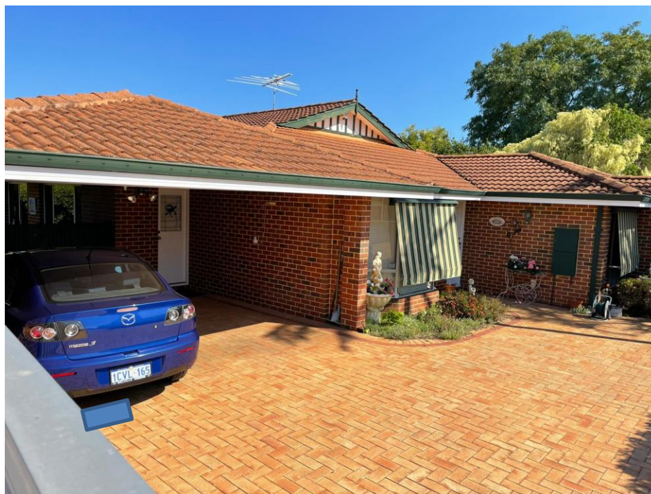
Figure 2. The proposed retaining wall will abut the existing carport of the neighbouring northern property – 7A Chesson Street, Alfred Cove – and will not directly abut any habitable spaces.
