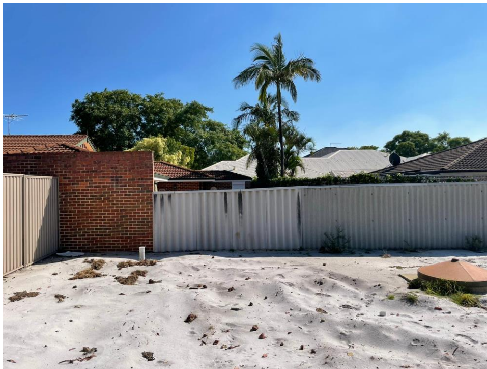
Figure 1. View of the rear of proposed Lot 700 (northern boundary). The subject retaining wall will abut this boundary.
