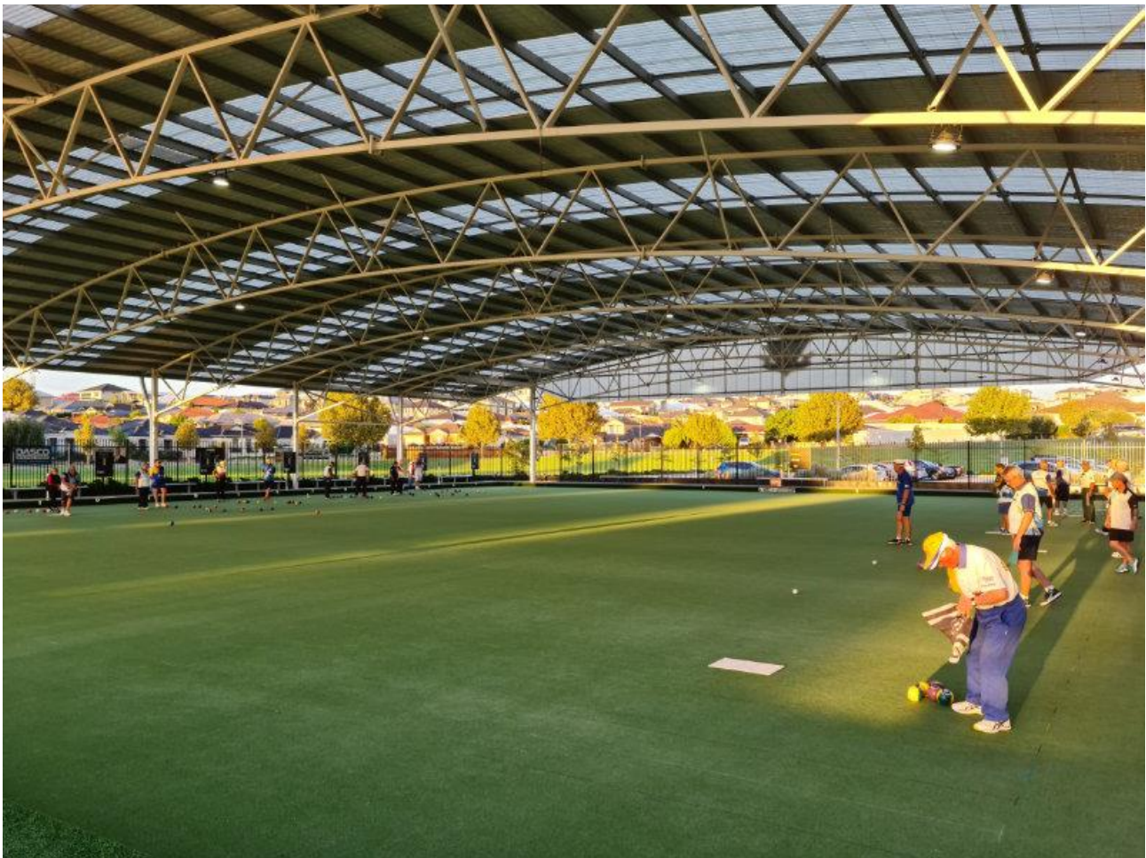
Figure 2 – Steel undercover area
