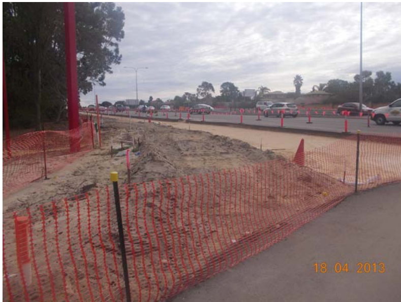
Image 2 – Looking west along South Street
