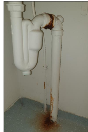
Ref # - 04 | Rusted drainpipe in toilet
