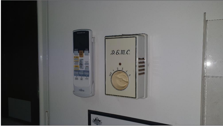
Ref # - 09 | Old fan switching to be tested
