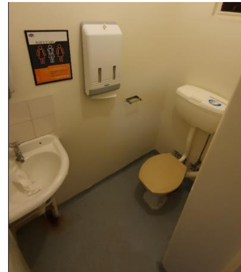
Ref # - 08 | Toilet and basin
