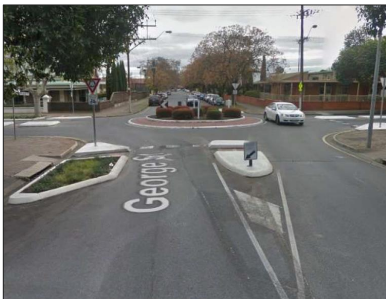
Figure 5-2: Radial Roundabout (George Street/Beulah Road, Norwood, SA)
