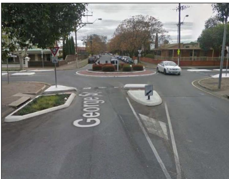
Figure 5-2: Radial Roundabout (George Street/Beulah Road, Norwood, SA)
