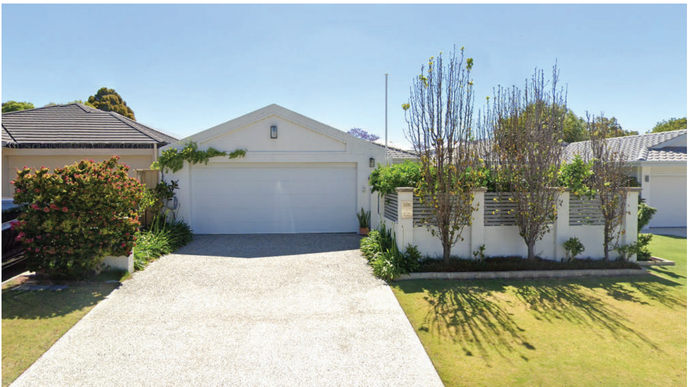
Figure 6. 30 St Michael Terrace, demonstrating local design features
