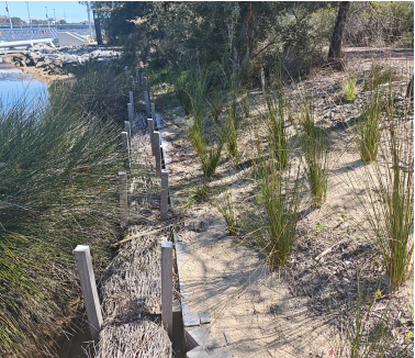
EXAMPLE OF RETAINING TIMBER WALL WITH BRUSHWALL WAVE DEFLECTOR
