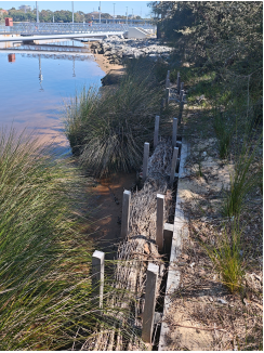
EXAMPLE OF RETAINING TIMBER WALL WITH BRUSHWALL WAVE DEFLECTOR
