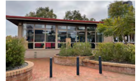
Canning Bridge Library exterior
