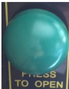
Press green button to exit the building.
