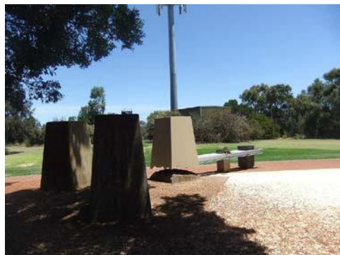
Guy anchor blocks for aerial mast.
