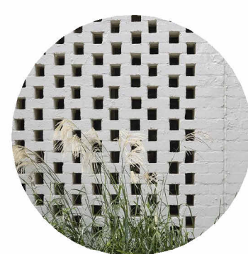
HIT AND MISS BRICK WALL INFILLED WITH GLASS BLOCK
