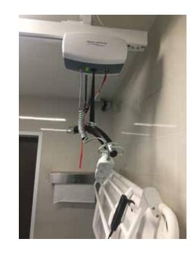
6. Emergency lowering strap can be used to lower a person in an emergency.
