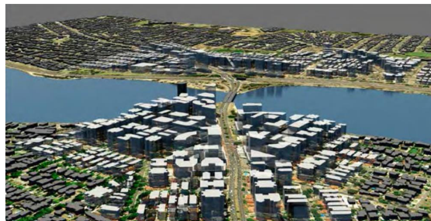
Figure 6 – Final stages of build out of western quarter (Source: CBACP Part 2)
