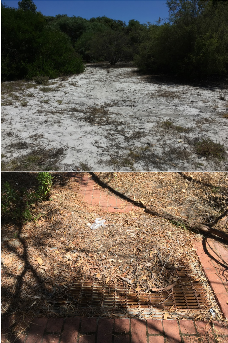
Figure 11.1-2: A) Sandy area in Trevor Gribble Park compensation basin where planting is recommended; B) grate in Trevor Gribble Park compensation basin with leaf litter and sediment sitting on top.
