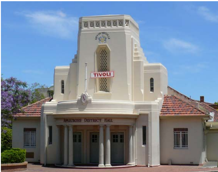
Heritage listed Applecross District Hall
